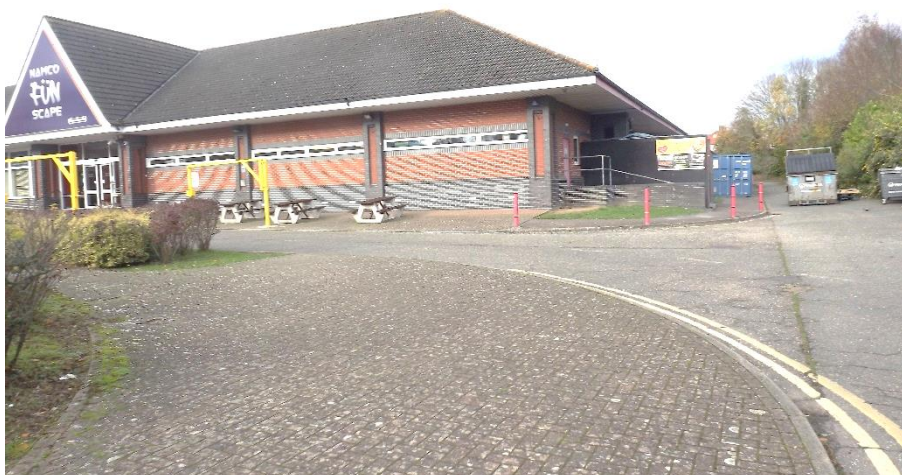
Building to be demolished and access to car park
