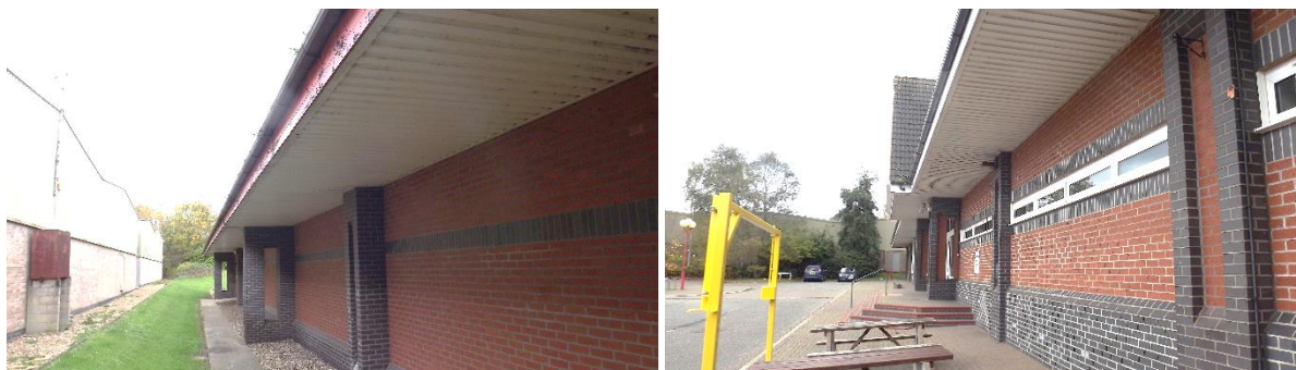
Figure 5- View of west elevation (left) and overhanging roof eaves (right)
