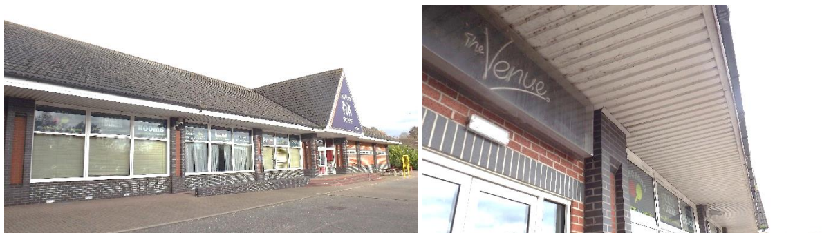
Figure 4- View of south elevations
