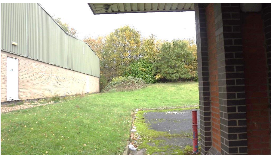
North-west corner of the site
